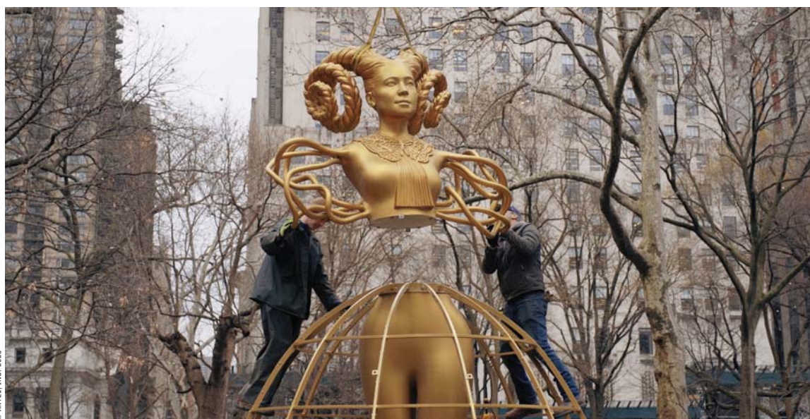
Left: Installation in process of Shahzia Sikander's Havah . . . to breathe, air, life (2023); Production still from the Extended Play film "Shahzia Sikander: Melting Boundaries"
